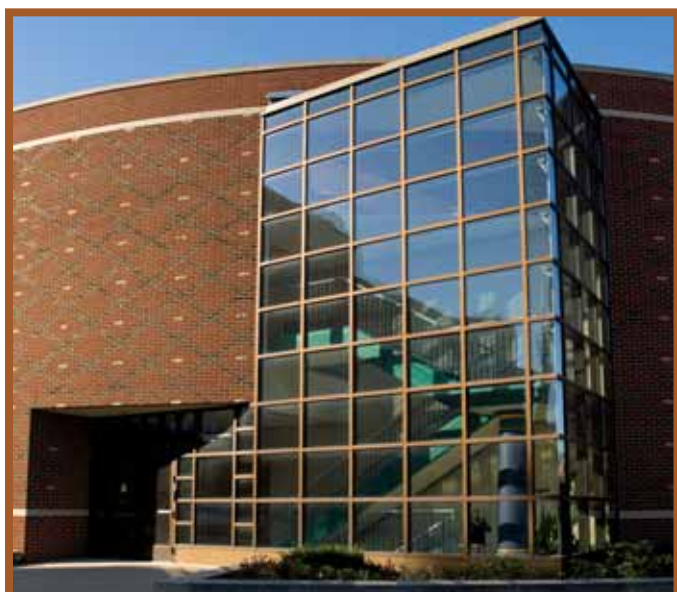
Purdue University has installed Sloan's UPPERCUT® dual-flush Flushometers in two administrative buildings on the West Lafayette, Ind., campus.
