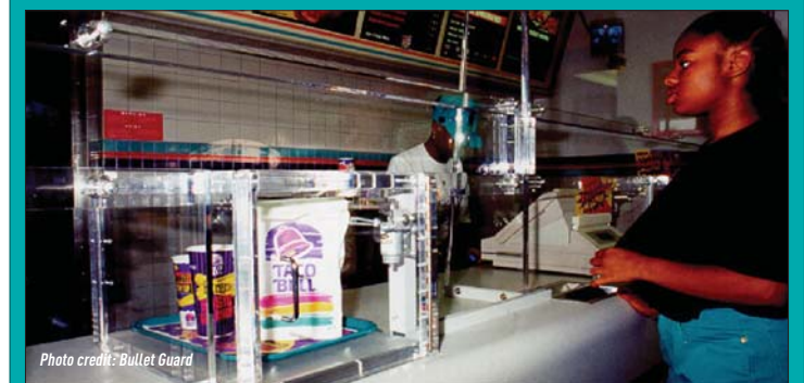
Fixed Counter Enclosure with Interlock Package Exchange and Continuous Voice Port
