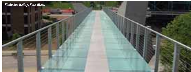
Photo Joe Hailey, Ross Glass Holmberg Pedestrian Bridge, Chattanooga, Tennessee The use of laminated glass with advanced polymer interlayers allowed strength and transparency in this key waterfront redevelopment project. Architect: Derthick Henley & Wilkerson Architects, Chattanooga
