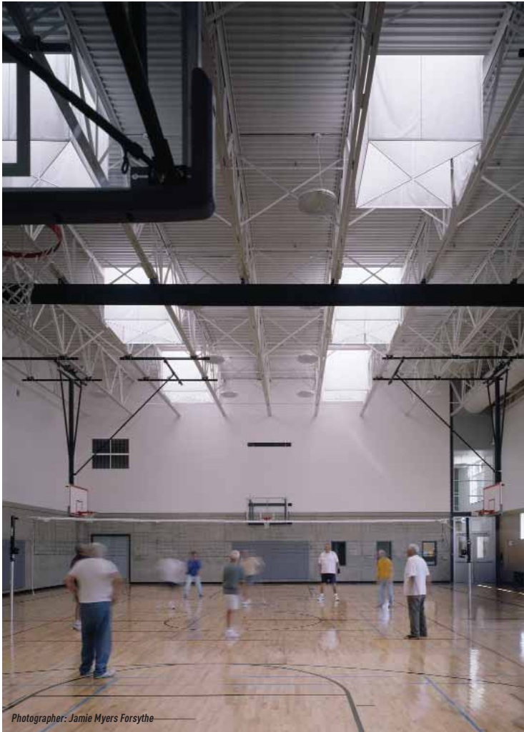
Southwest Community Center Gymnasium, Seattle, WA: This gymnasium uses fabric skylight baffles to diffuse glare and make electric lighting unnecessary during daylight hours. Architect: Weinstein A|U
