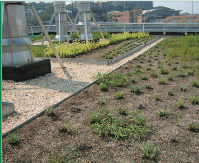
Staten Island Ferry Terminal—St. George Terminal, Staten Island, NY • Architect: New York office of Hellmuth Obata + Kassabaum This one-quarter acre extensive green roof provides rainwater collection for irrigation and stormwater retention.
