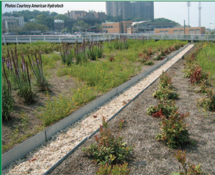
Staten Island Ferry Terminal—St. George Terminal, Staten Island, NY • Architect: New York office of Hellmuth Obata + Kassabaum This one-quarter acre extensive green roof provides rainwater collection for irrigation and stormwater retention.
