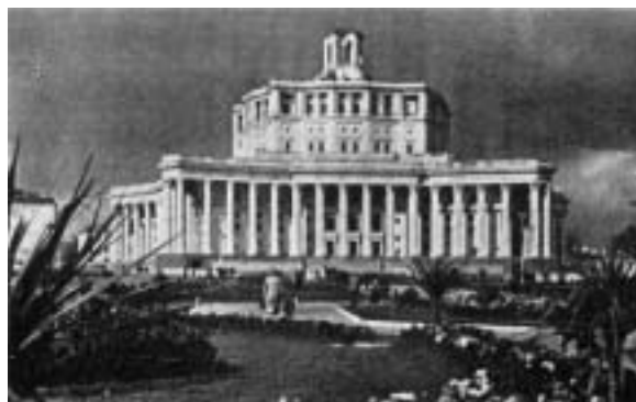
Central Theatre of the Soviet Army. Architects K. Alabyan and V. Simbirtsev. The Red Star shaped plan was approved.
