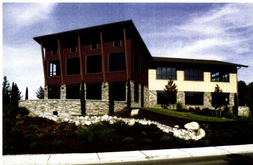
Installation of a manufactured stone system requires the choice of a believable color palette and careful placement of masonry units on exterior walls and building facades to maximize the illusion of natural stone.
