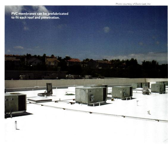
and stabilizers into single-ply membranes, which prolong material life. At this point, the single-ply roofing industry has a proven performance record of more than 30 years.
