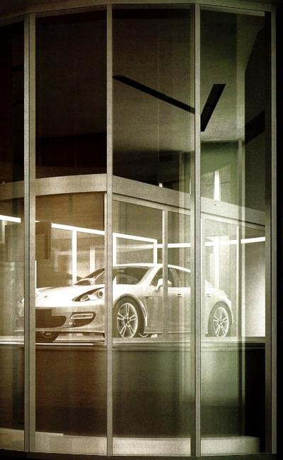
2 HOUR FIRE RESISTIVE **GLASS ELEVATOR ENCLOSURE** WITH SUPERLITE II-XL 120 IN GPX CURTAIN WALL FRAMIN
