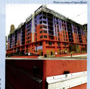
There was 150,000 square feet of self-adhered, water-resistive, vapor-permeable air-barrier sheet membrane installed on The Banks Phase II mixed-use building (top). Shims used under horizontal cladding attachment components create a 14-inch rainscreen cavity, allowing for unimpeded vertical drainage of moisture away from the building envelope (bottom).
