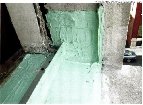
Liquid flashing installation at window opening—single material and installation operation.
