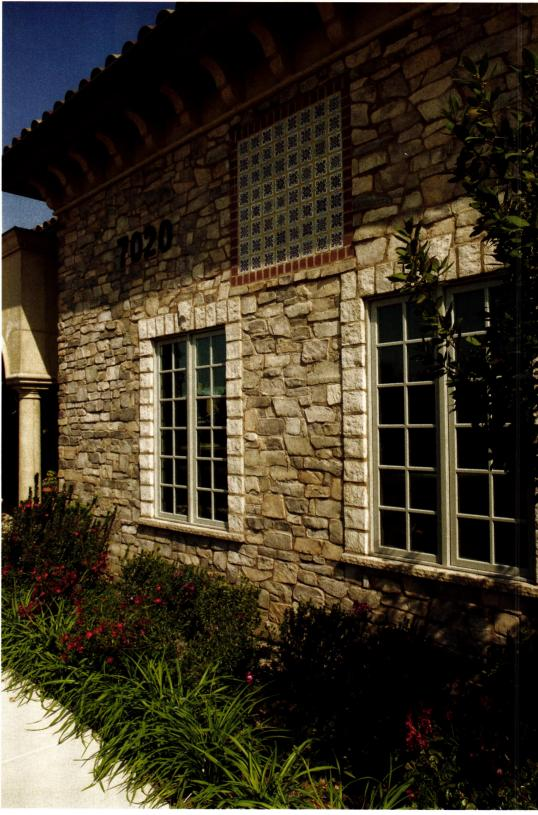
Foundation treatments that obscure the required termination of manufactured stone above grade can include a bed of stones placed adjacent to the wall along with a landscape area beyond that can screen the transition.
