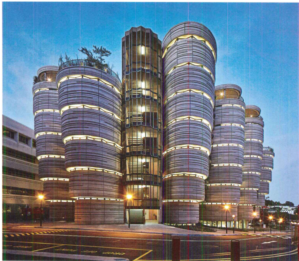
The Learning Hub for Nanyang Technological University in Singapore opened early in 2015. Heatherwick worked with local architects, CPG Consultants, on the design for the poured-concrete cluster of eight-story zucchini-shaped towers.
