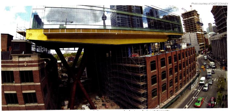
Architecturally exposed structural steel used on buildings of all types can now also be true design statements due to the availability of cast steel connectors in the U.S. and Canada.
