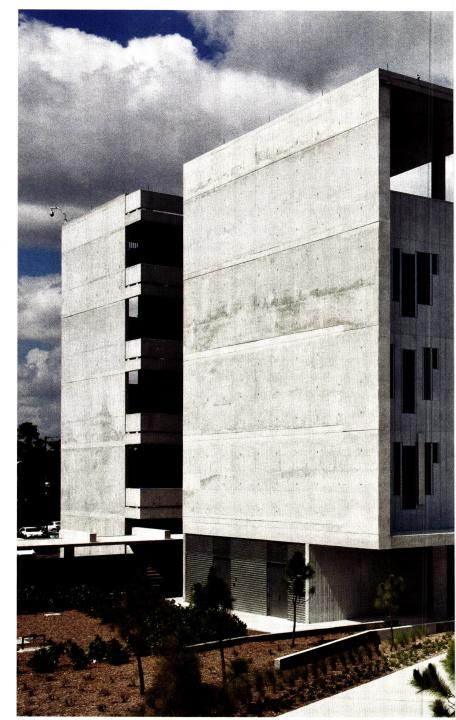
plane into something that almost appears to float. Flat-plate concrete construction allows floors to rest directly on columns, eliminating the need for beams and simplifying the building's visual expression.
