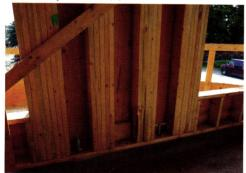
With five- and six-story wood-frame buildings, greater height creates a need for more structural framing, especially at lower floor levels. Stud packs of built-up stud columns may be utilized to meet seismic and gravity loadcarrying requirements. In many of these walls, the use of exterior-insulated assemblies may be more efficient than insulating stud cavities.
