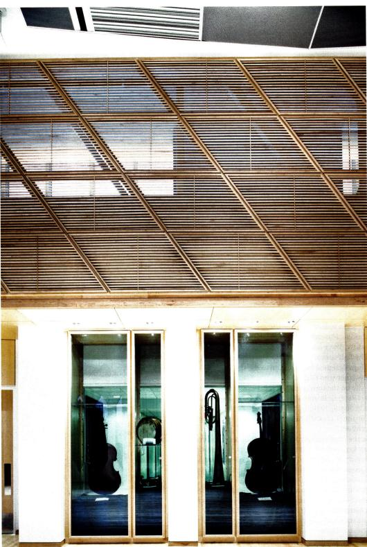
reinforce the diagonals of the trusses. The composition creates a delicate veil on the interior that lets in filtered sunlight during the day through the new clerestory's insulated glazing units. After dark, the transparent box becomes a lantern, with the area below in use at all hours of the night, as both an informal rehearsal area and a recording room.
