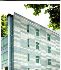
ABOVE: Fiber cement architectural wall panels are an advanced product compared to residential fiber cement siding and offer a full range of performance, aesthetic, and cost solutions.
