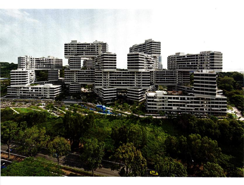
left OMA, that threatens to further pigeonhole the architect. It is a breathtaking one, made up of 31 six-story rectangular blocks that appear woven, and are arranged on top of each other at angles. The flush, white-painted concrete facades are occasionally interrupted by slender horizontal balconies, from which greenery will cascade as it grows. The building snakes around and through its roughly rectangular 20-acre site like a line of toppled dominoes.
