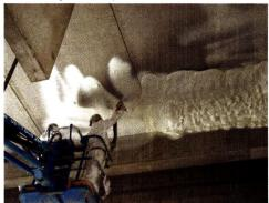
Open cell, low-density spray foam insulation is applied in a continuous application against wall sheathing or roof decking.
