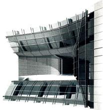
SCULPTED AND SHAPED The tower's envelope includes four inlets or ducts (above), each containing a vertical axis wind turbine (left). CFD modeling (bottom) helped designers shape the ducts to accelerate the speed of the wind rushing through them and therefore increase the electricity-generating potential of the turbines.
