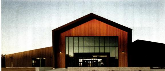
NATURAL AND OFFICIAL In the barnlike assembly hall used for both military and community functions (above). slatted screens of Douglas fir conceal HVAC equipment, acoustical panels, and skylights. The assemblage of sheds (right, top) is clad in wood and metal. The glazed southwest end of the assembly hall (bottom right) opens onto a terrace.
