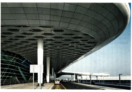
SPACE ODYSSEY Although vast, the departures hall is given definition by its undulating ceiling, and scale by freestanding "trees" that supply air and electric light (previous spread). A canopy at the terminal's south end extends to an oval groundtransportation center (left and above). As in the departures hall, folded-metal panes form hexagonal openings in the soffit of the canopy.
