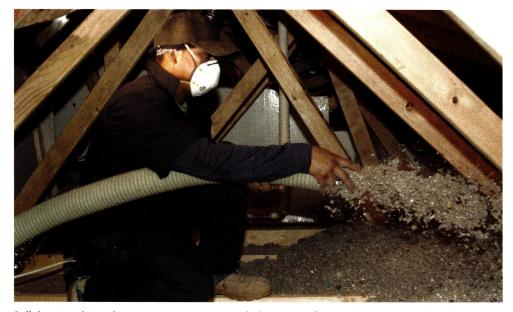
Cellulose insulation has a post-consumer recycled content of up to 85 percent and can be more effective and economical overall than other insulations with the same R-value per inch.
