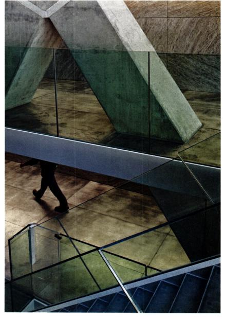
GOOD BONES As it has done in large Asian projects like the CCTV tower in Beijing and the Shenzhen Stock Exchange, OMA exposed the building's structural frame on the inside and used it as an important element in spaces such as the stair hall for restaurants and bars (above). Generous balconies on the residential section of the project provide city views from the apartments (top).
