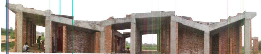
The architect was inspired to design the brick screen after a visit to the westernmost areas of China, including Kashgar in Xinjiang province. The screen helps keep the house cool in summer and warm in winter (above). An angled concrete roof collects and stores rainwater and provides a place to dry food (left and below left). Two women live in the house, which is also used for a women's weaving cooperative (below).
