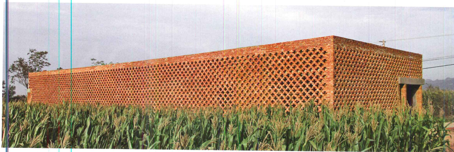
The architect was inspired to design the brick screen after a visit to the westernmost areas of China, including Kashgar in Xinjiang province. The screen helps keep the house cool in summer and warm in winter (above). An angled concrete roof collects and stores rainwater and provides a place to dry food (left and below left). Two women live in the house, which is also used for a women's weaving cooperative (below).
