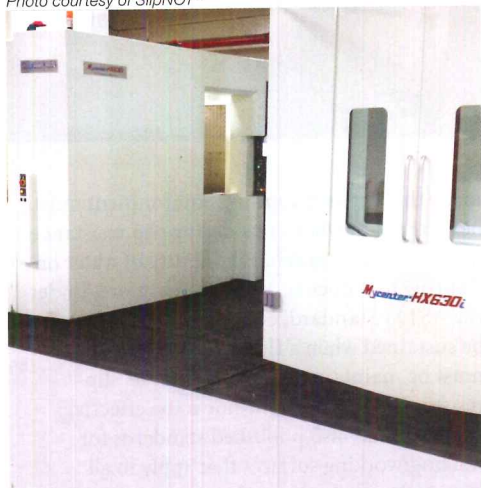
Bremen Castings, Inc. installed slip-resistant steel plates around their CNC machines where oil and coolant collect on the foundation pit. This provides a safer work surface for their personnel.
