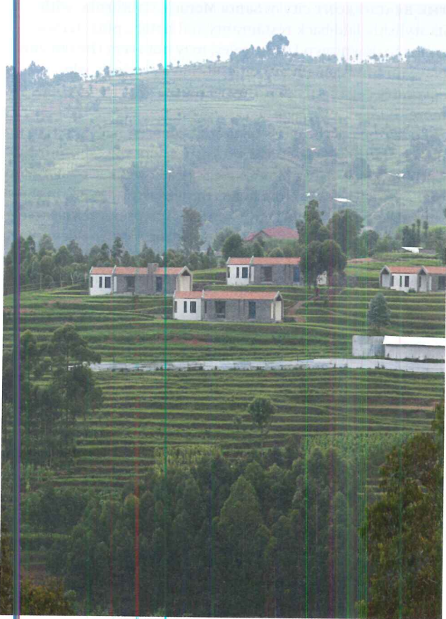
HEALING HILL Rather than excavating, the architects stepped the houses down a hill to have a light touch on the topography (above). Visitors enter the site from the south. Each house has its own courtyard gardens; these are important spaces for Rwandans to gather with friends and family (opposite). MASS recruited local artisans to fabricate the custom interior furnishings on-site; reclaimed-metal light fixtures, woven papyrus chairs, and cypress and pine tables and desks can be found in each house (right, below, and below right).
