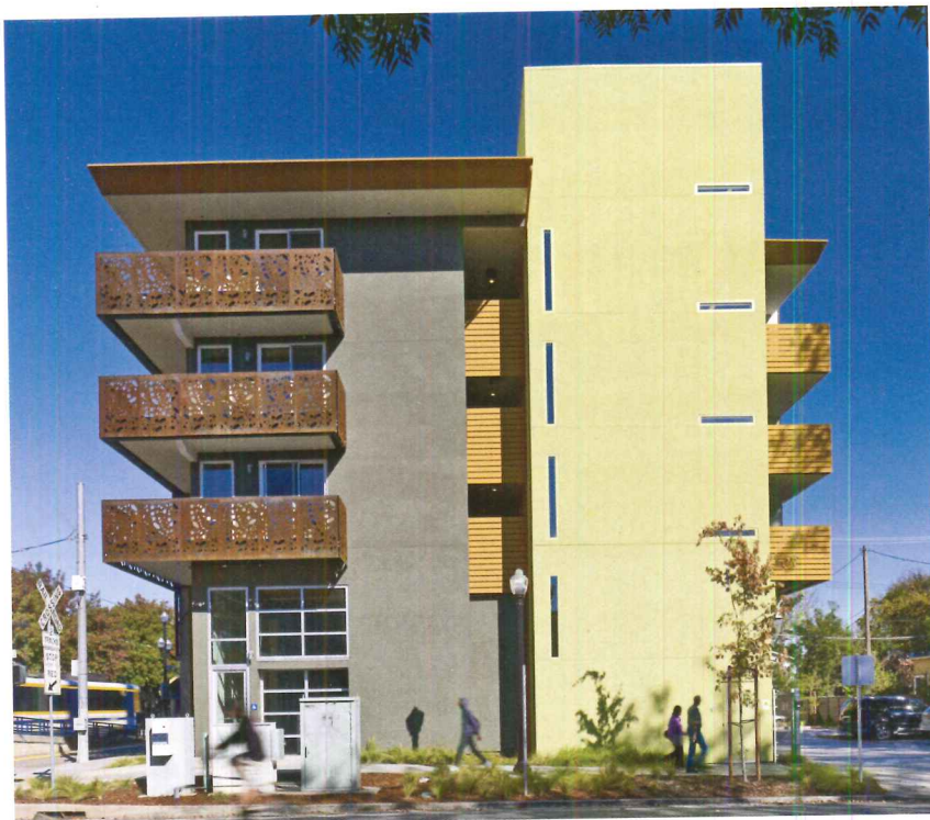
LINEAR AND LEAN As the southern-end elevation of La Valentina Station (above) shows, the long and narrow residential complex is girded with balconies. The amenity gives a sense of spaciousness (right) to the apartments in the wood-frame and concrete-deck four-story structure.
