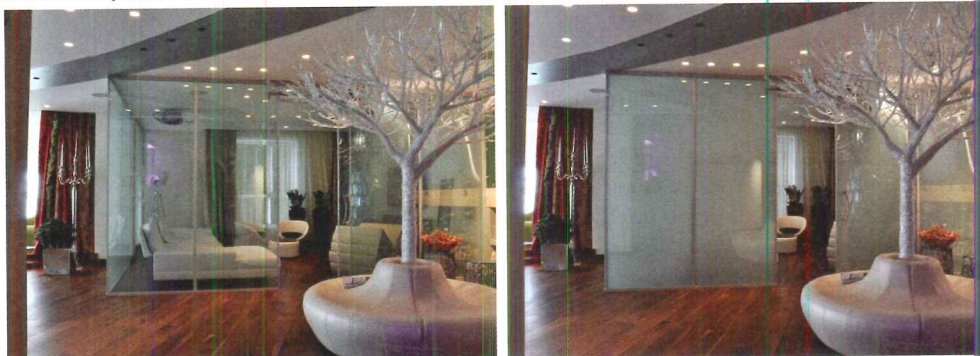
With switchable or “intelligent” glass technology, glass finishes go from clear to opaque.
