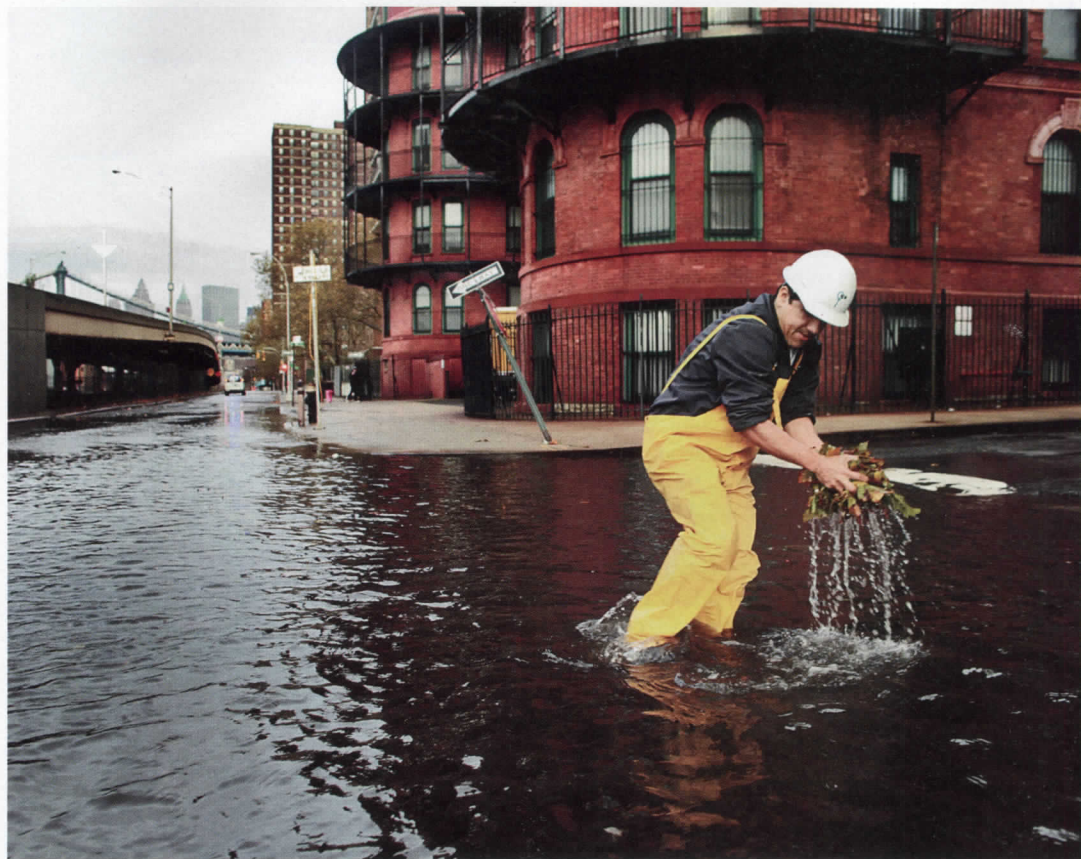
A New York City worker clears a sewer drain in Lower Manhattan after Superstorm Sandy.
