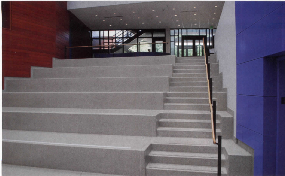
Terrazzo requires minimal maintenance and has fewer joints than other flooring types. The material also provides for good IAQ by reducing potential locations for mold to develop and grow.
