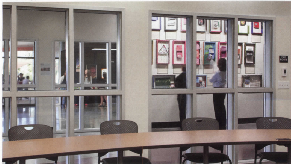
Fire-rated glass and framing systems have been used by architects to create visually appealing glass separations that use robust, fire-protective and fire-resistive glass.
