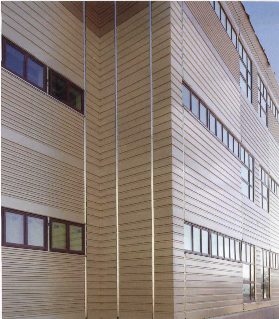
This middle school received a 3-inch insulated panel system, which provides an R-value of 21 on top of the insulating value of the wall beneath, which helps schools endure harsh winters and save energy without requiring excessive façade maintenance.
