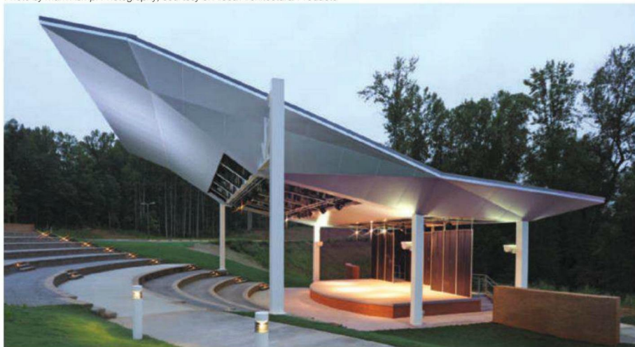
The canopy at the Piedmont College Arrendale Amphitheater, Demorest, Georgia, was sculpted from aluminum composite material to reflect the natural environment bordering the site. Architect: Armentrout Roebuck Matheny Consulting Group.
