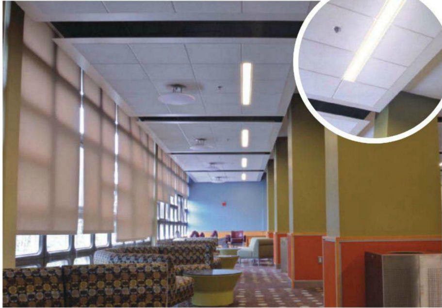
Linear LED luminaires provide soft lighting for Boston University Rich Hall residence in Boston, Massachusetts.
