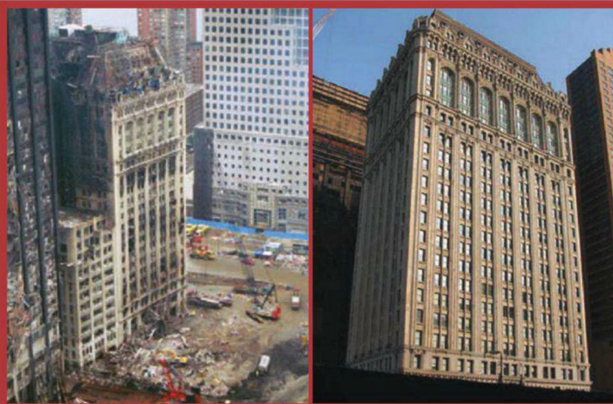
Demonstrating the resilience of CMU, the West Street Building by Cass Gilbert was reopened in 2005 after being damaged by the World Trade Center collapse and a five-day fire in 2001.
