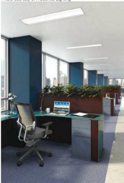
The IESNA recommends that an open-plan office maintain 400 lux (40 footcandles) at the working level.
