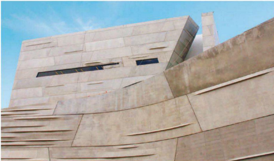
Precast concrete façade cladding on the new Perot Museum, affords durability, low maintenance costs, and high thermal mass, among other benefits.
