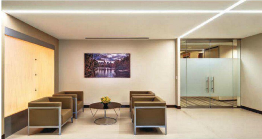
Continuous-run linear LED luminaires were specified in custom lengths for the Chapwood Capital Investments office in Dallas, Texas.
