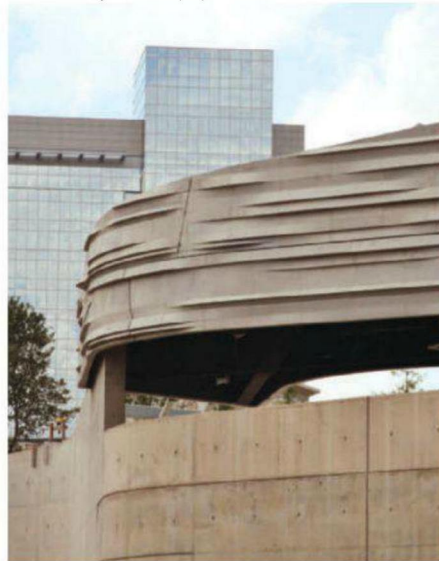
The concrete mixes for the project included up to 51 percent slag in core walls, and 50 percent fly ash in piers, columns, and slabs.
