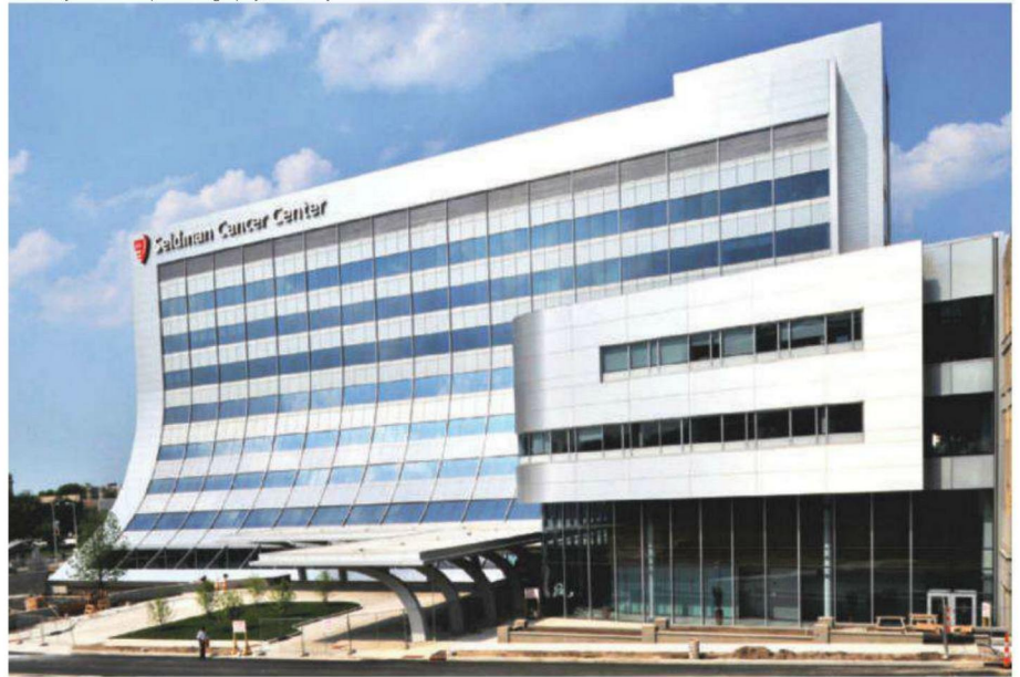
The 10-story, 375,000-square-foot Seidman Cancer Center in Cleveland, Ohio, features 59,000 square feet of brushed aluminum composite material on the exterior and the interior building fascia, soffits, and parapet panels. Architect: Cannon Design.
