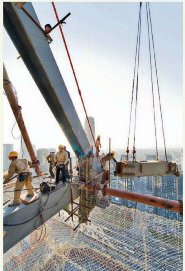
BALANCING ACT Countering criticism that its complex design is wasteful, Arup and OMA say the building required no more steel than a conventional structure of its size. The Chinese contractor erected the two angled towers (top photos) and then the cantilevers that were connected to each other early in the morning of December 8, 2007 (above).
