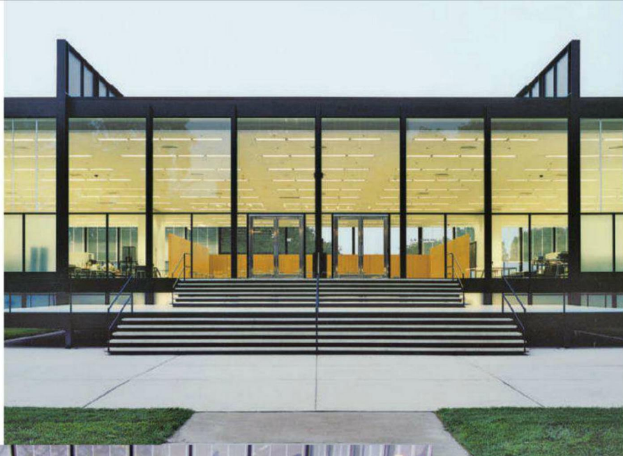
S.R. CROWN HALL, ILLINOIS INSTITUTE OF TECHNOLOGY, CHICAGO. MIES VAN DER ROHE, 1956. RENOVATED BY KRUECK+SEXTON ARCHITECTS, 2005.
