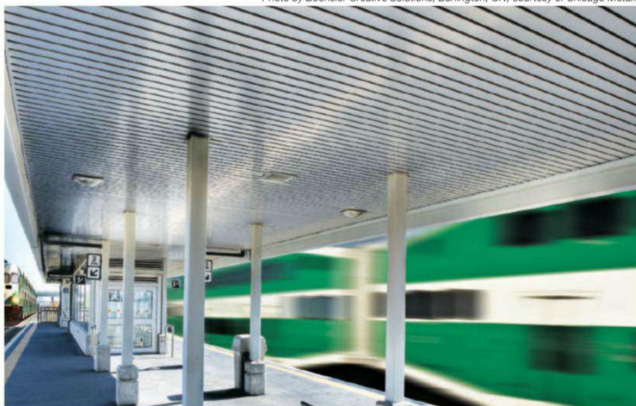
Interior and exterior linear metal ceilings provide visual continuity and performance at a Go Transit Station in Brampton, Ontario, Canada. Consulting engineer: R.J. Burnside & Associates Ltd.
