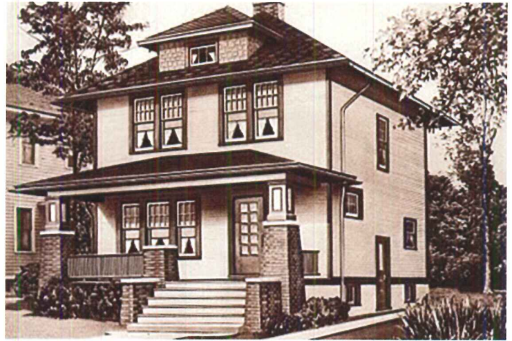
The Fullerton Kit house, as pictured in a 1920s Sears, Roebuck “Modern Homes” catalog. Houses like this reassure us and reiterate what has long been a part of our lexicon.
