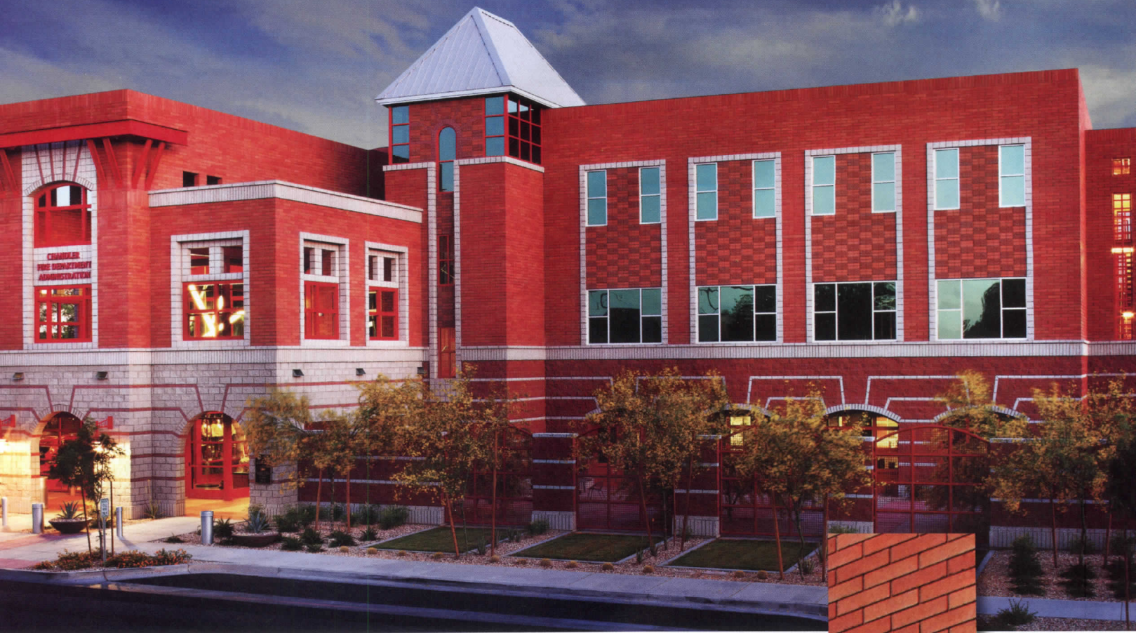
-Project: Chandler Fire Administration Building, Chandler, AZ.
