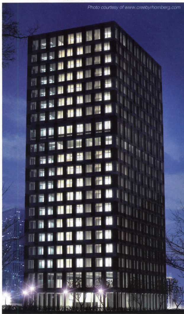
The 30-story LifeCycle Tower to be built in Dornbirn, Austria features a hybrid construction system based on wood.
