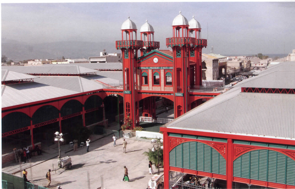
Architect John McAslan has revived the Iron Market (above), which suffered extensive damage during the 2010 earthquake (below).
