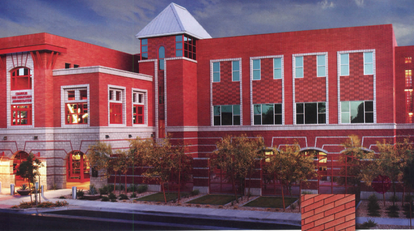
-Project: Chandler Fire Administration Building, Chandler, AZ.
