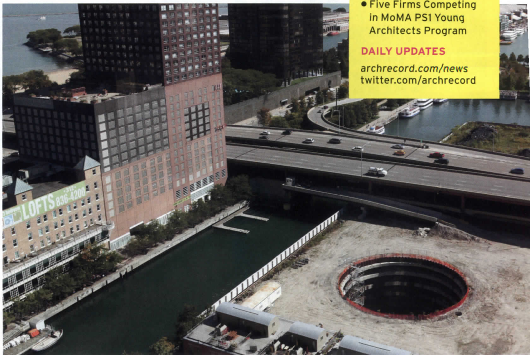
Numerous projects have been halted globally, including Calatrava's Chicago Spire, now a 76-foot-deep hole.
