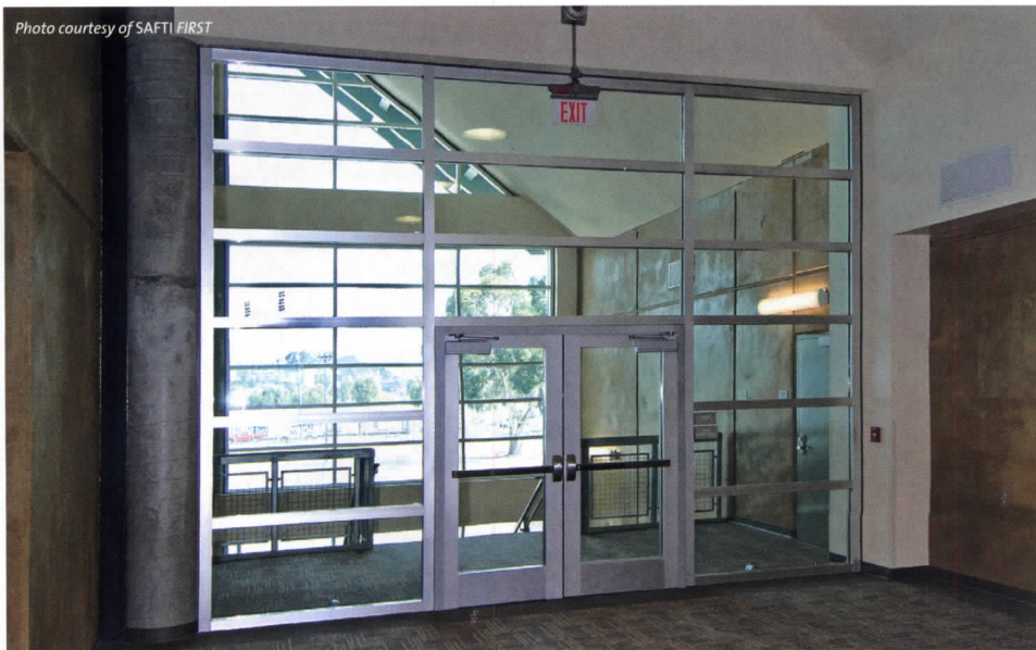
Fire-resistive glass assemblies can create a sense of openness, add natural lighting, and increase the visibility to safe pathways.
