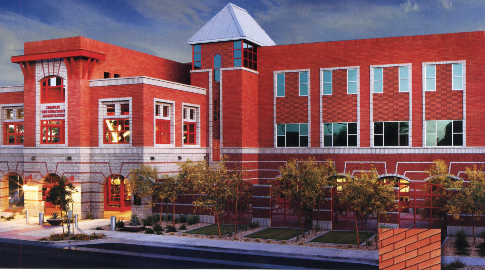
-Project: Chandler Fire Administration Building, Chandler, AZ.
