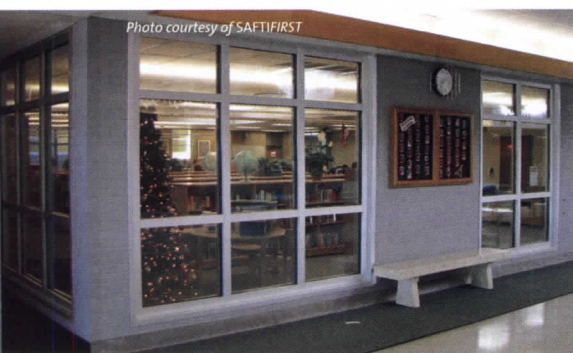
Stringent fire-safety criteria were met in the corridor designs at North Layton Junior High School.
