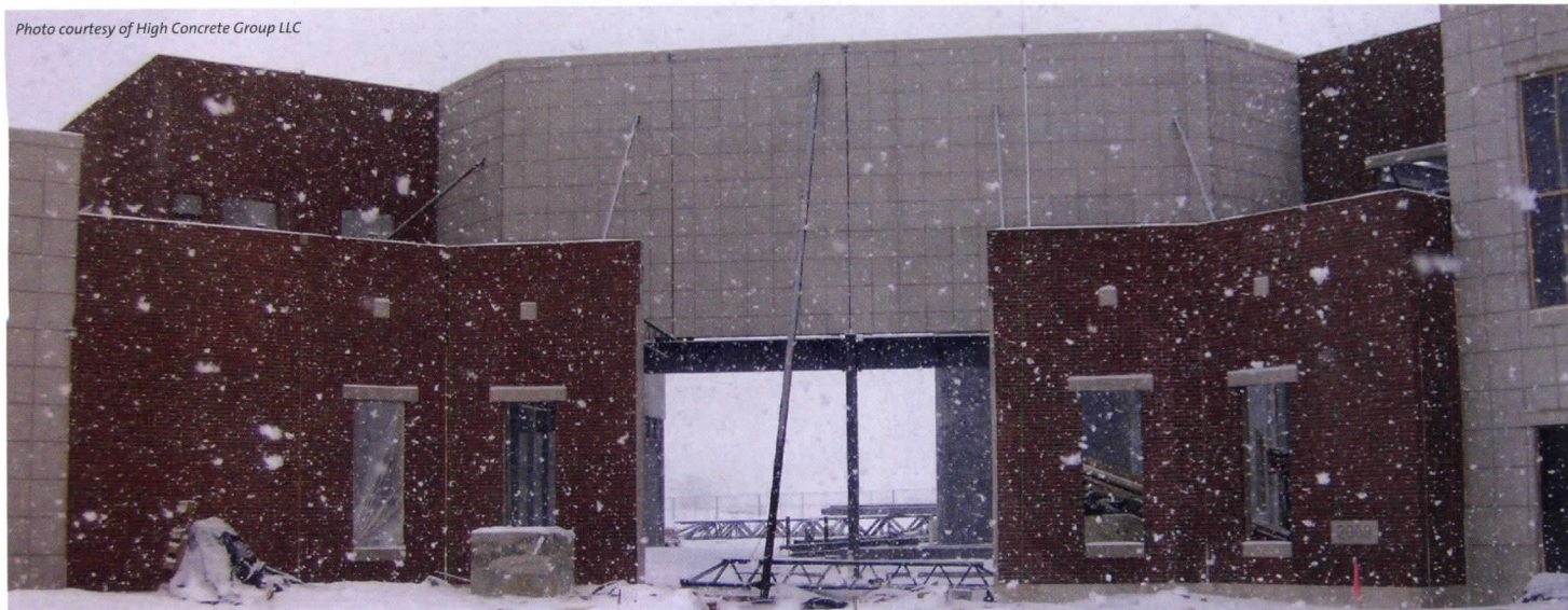
Precast concrete can be quickly erected even in the winter, as shown in construction photo of Willow Creek Elementary School in Fleetwood, Pennsylvania. Designed by AEM Architects Inc.
