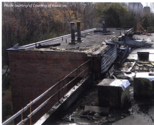
Roofing insulation stands up to an intense four-alarm fire at York University in Toronto, Canada. Noncombustible stone wool insulation prevented the fire from spreading, avoiding damage to property and possibly any human loss.
