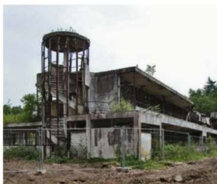
Located in Hilversum, the Netherlands, the Zonnestraal Sanatorium fell into disuse after World War II.
