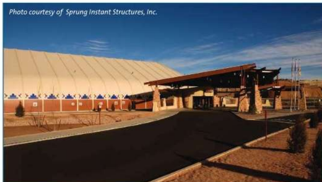
Photo courtesy of Sprung Instant Structures, Inc.
