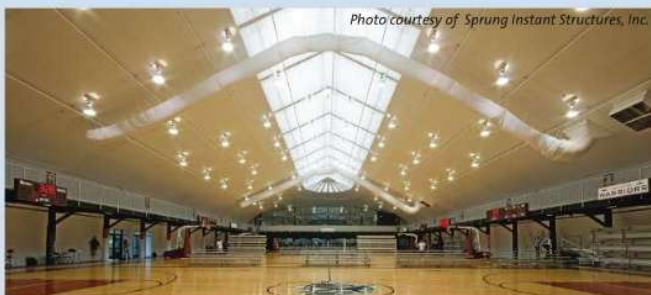
Photo courtesy of Sprung Instant Structures, Inc.
