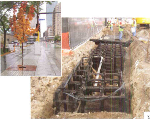
5 | PRODUCT Silva Cell Subsurface Tree Protection and Stormwater System MANUFACTURER Deep Root Partners deeproot.com
