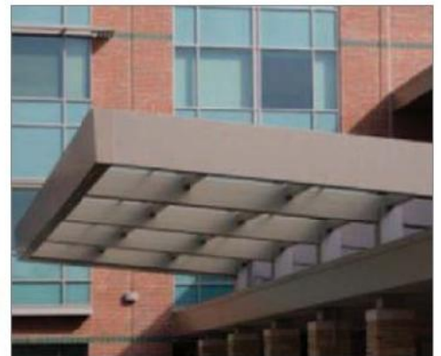
STAFFORD HOSPITAL STAFFORD, VIRGINIA Composite panel entrance canopy
