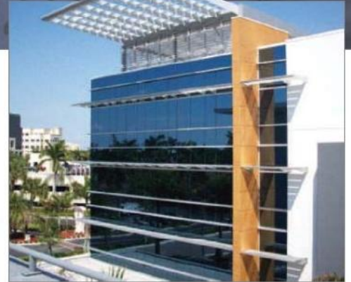
OFFICE BUILDING Boca Raton, FL Sunshade canopy & curtain wall sunshades
