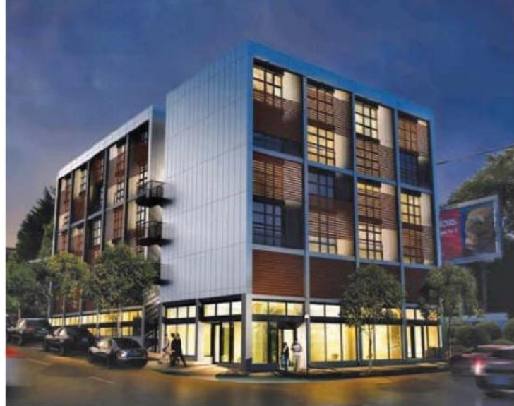
151 Lofts, Seattle, 2010 The design for this 18-loft-unit building includes 5,600 square feet of commercial space and features solar shading, green roofs, and natural ventilation.
