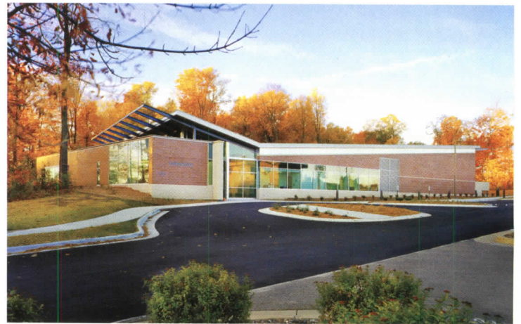
UW Cancer Center's plethora of windows allow for visual connections to its wooded site, as do meandering paths around the facility.
