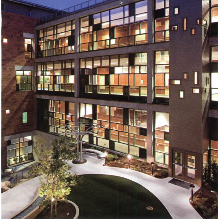
Dell's entrance tower acts as a landmark (opposite). The courtyards, most of which are accessible, serve as air intakes for the building (left and below).
