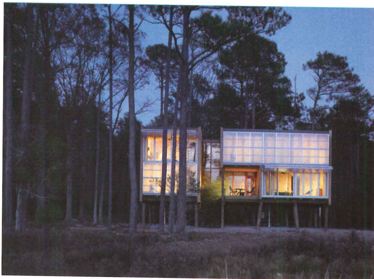
Mostly opaque on the three sides facing the woods (opposite), the house opens to the west (left) with views of the Chesapeake Bay.
