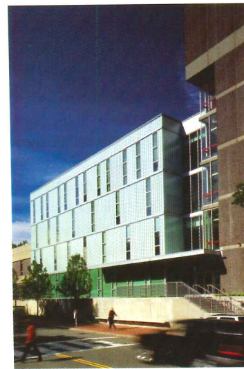
LWA recently completed this expansion of the Harvard Science Center.
