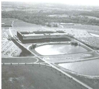
Ma Bell facility will be demolished.
