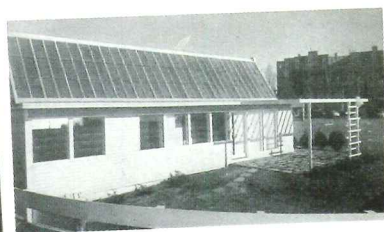
Another view of the house with "sun-measuring" gadgets called pyrheliometers evident on the eaves and peak (right) of the roof. They measure the intensity of solar radiation outside a collector tilted at the 57 degree angle or oriented vertically.
