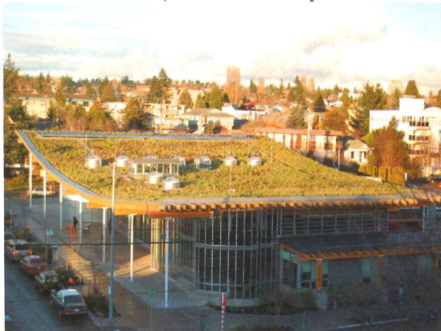
Ballard Library - Seattle, WA (2006 Green Roof Awards of Excellence winner)
