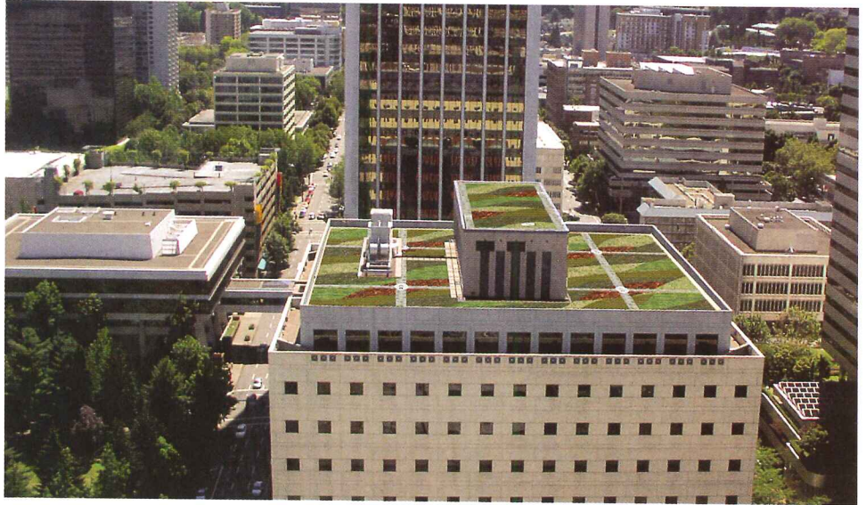
Michael Graves's Portland Building will soon have a green roof as the result of a local resolution passed earlier this year. Officials will monitor how effectively the installation mitigates storm-water runoff.
