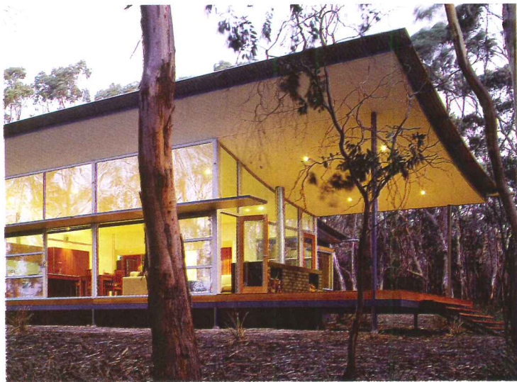
Tasmania's Walla Womba Guest House by 1+2 Architecture (2003), raised on a steel frame, treads lightly, preserving the woodland's natural drainage patterns.
