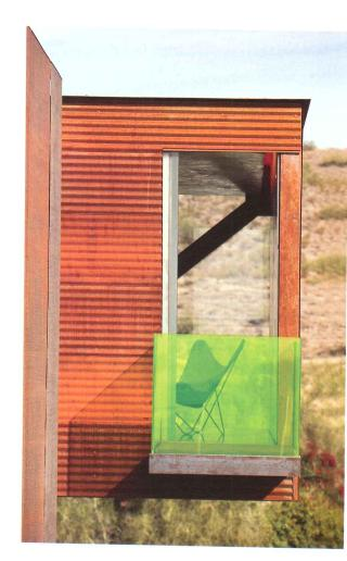
Phoenix sprawls, and the bedroom to the north, facing the unpopulated mountains. The 24-foot-long bedroom wing cantilevers 12 feet to the east from the house's 12-foot-wide base to include a home media center. The base, containing a library and studio, is partially enclosed by sloping concrete foundation walls, and depressed slightly below grade along the hill's 5-degree incline. To the south, the studio opens onto an enclosed outdoor patio and, beyond that, a 14-inch-deep pool.
