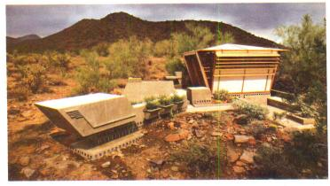
Trevor Pan stretched "sunbrella" fabric over wood beams to create a sleeping shelter at Taliesin West. At the corners, open louvers provide natural ventilation.
