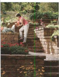
VERSA-LOK is the industry's original solid, pinned segmental retaining wall system, offering unequalled design versatility and ease of installation. VERSA-LOK is available in attractive split-face and vintage weathered textures, and readily accommodates soil reinforcement to build walls 50-ft. or taller. VERSA-LOK Mosaic combines random-pattern beauty with VERSA-LOK brawn. Email versalok@versalok.com
