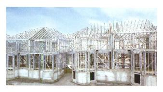
individually or as a complete engineered framing system. After the components are delivered to the job site ready to install, small crews can frame a home in a fraction of the time it takes using traditional methods. Steel components are dimensionally more stable than wood and resist fire, mold growth, and termites. USG, Chicago. www.usg.com circle 215
