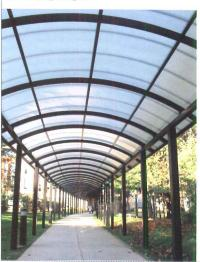
CPI provides single source responsibility for entire structure from the ground up. CPI's new Clearspan design for translucent canopies and walkway covers eliminates the horizontal cross beam and offers an economical, functional design with unequaled aesthetic appeal. Clearspan provides an excellent shelter and gives an open-air feeling by allowing natural daylight through to light up the area below.
