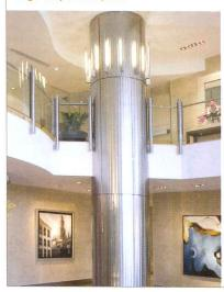
GageMetal®: An innovative collection of 16 designs suitable for walls, elevators and column covers. Standard sizes 48-in. by 96/120-in. with available thicknesses from .025-in. aluminum to 16 gauge stainless steel. Custom design and collaboration is available. Email gage@centurytel.net
