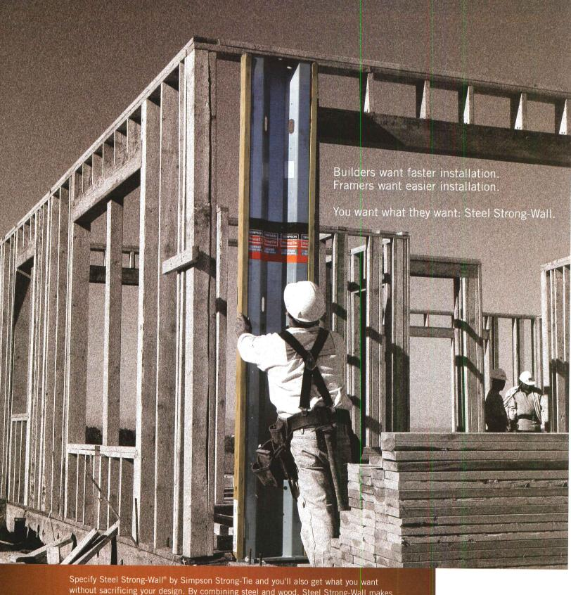
Specify Steel Strong-Wall® by Simpson Strong-Tie and you'll also get what you want without sacrificing your design. By combining steel and wood, Steel Strong-Wall makes it easy to achieve high loads in narrow spaces. Steel Strong-Wall is available in five widths from 12 inches to 24 inches and heights ranging from 7 feet to 13 feet. For more information on how Steel Strong-Wall can work for you, visit us at www.strongtie.com or call 1.800.999.5099.
