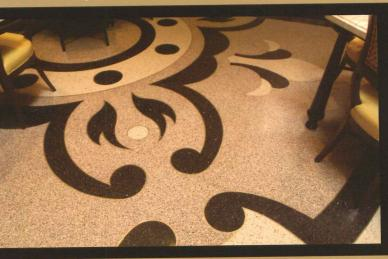
This dining room is highlighted by a terrazzo floor, which incorporates three earth tone colors, separated by ¼" brass dividers fabricated into fleur-de-lis designs of swirls, circles, and kite shapes, with all brass intersections mitered. All of the brass design work was fabricated on site from a small-scale hand drawn sketch, which was provided by the architect. The designs continue through the curved steps, which were cast in place, with a coping type radiused nosing.
