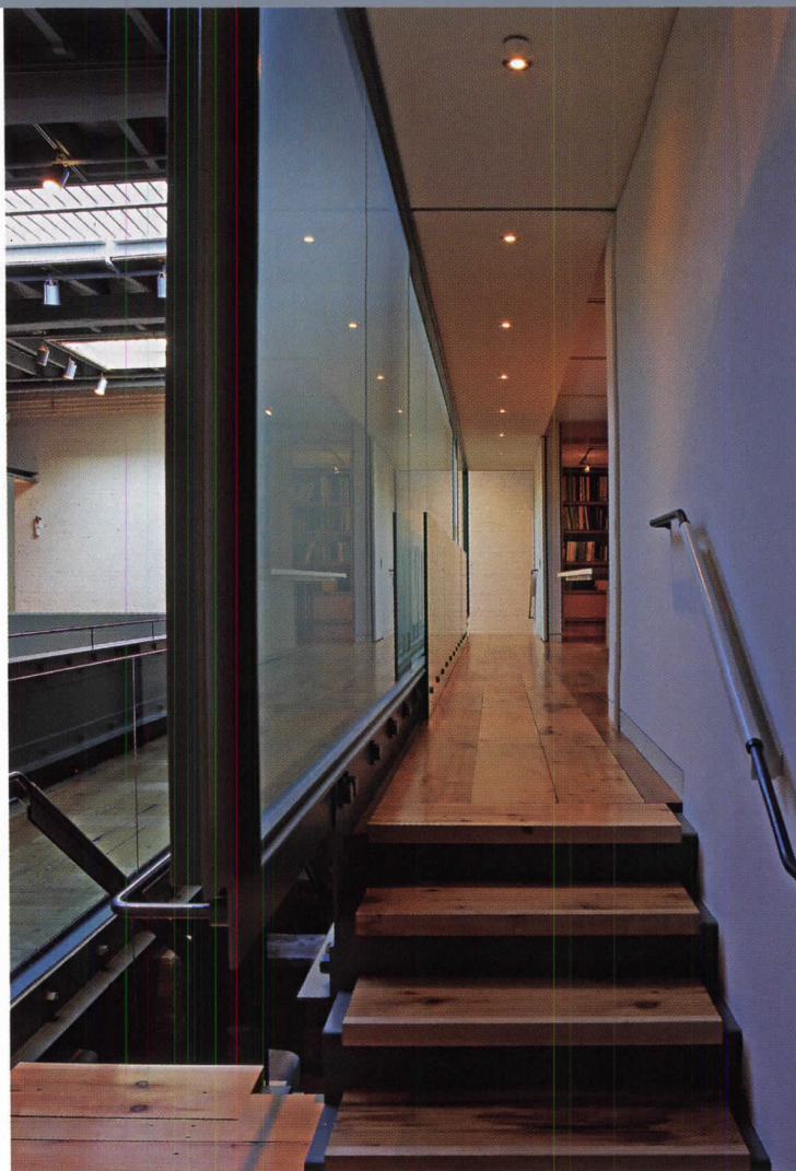
A new steel staircase with recycled wood treads is centered between massive brick archways to heighten
