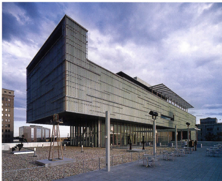
At the Shaw Center, the facade's glass channels (above) vary in size and shape to create depth and complexity. They also act as a rain screen.
