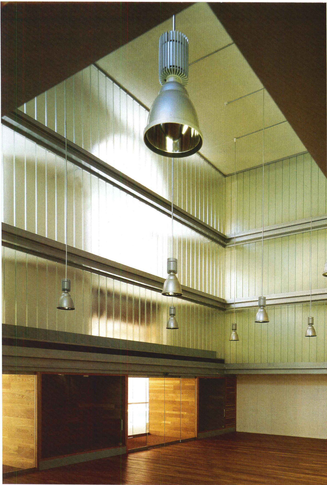
The library's lobby (left) is a three-story volume ringed with the same U-glass used on the exterior of the buildings.
