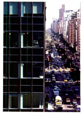
Whereas the wiredglass spandrel pan were originally divid into two parts with full mullion, now a nonfunctioning mul lion (above and left is applied to the pa els. The environmen codes for energy us were waived so that the same singlepaned glass could b installed.
