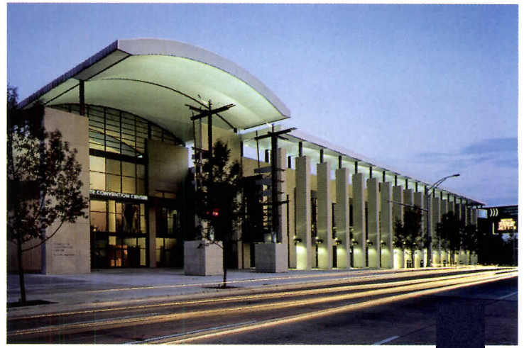
Charlotte Convention Center Charlotte, North Carolina, 1995
