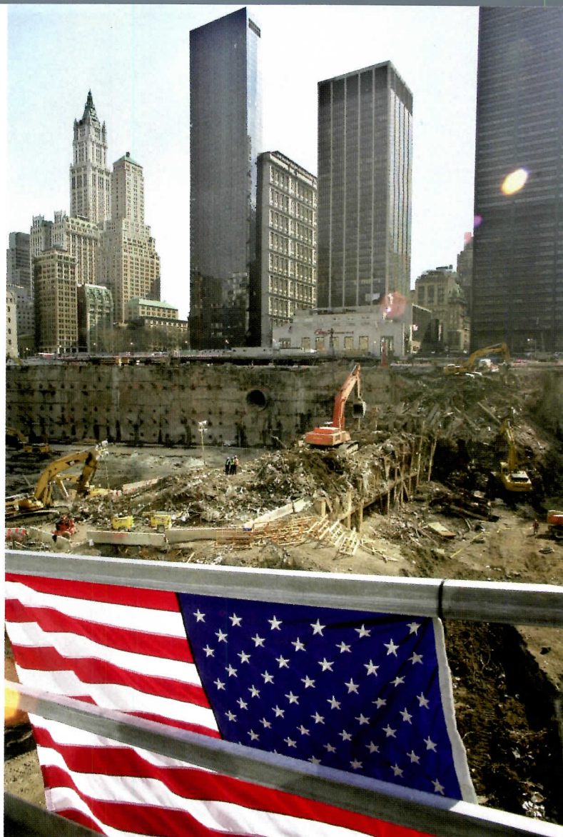
Heavy equipment digs into the last mound of debris at the WTC site in early March.
