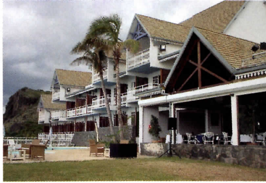
An impregnated oil protects Soveco shingles from insects and fungus.
