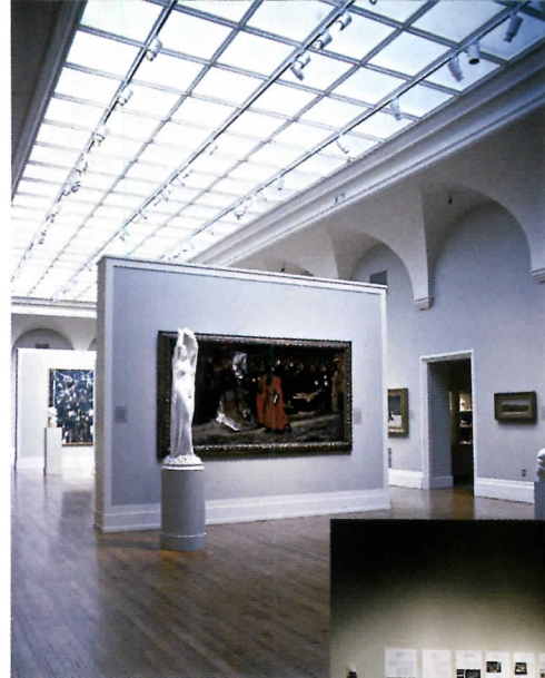
Painted over in the 1970s, the main gallery's laylight has been fitted with new laminated glass and a UV-absorbing interlayer (left). A furniture exhibition is lit by PAR30 and MR16 track fixtures (below).
