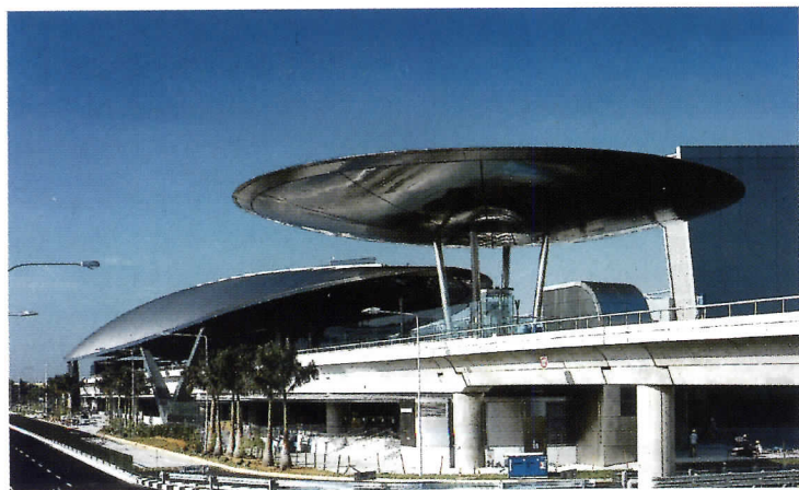
A jaunty, stainless-steel hat salutes passengers at the Expo Station on Singapore’s new city-to-airport rail line. The architect is Foster and Partners.
