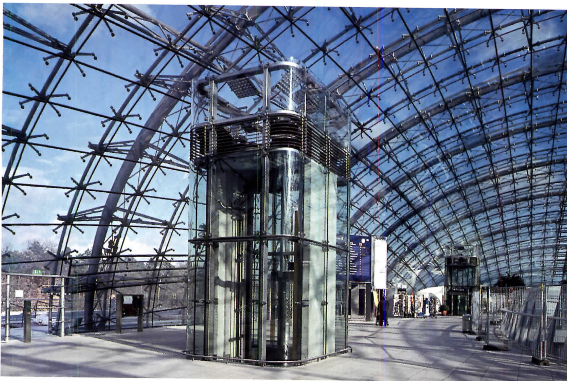
Tubular ribs frame the ticketing-level bubble (above) from the exterior (right), supporting armatures that attach glass by bolt-through connections.
