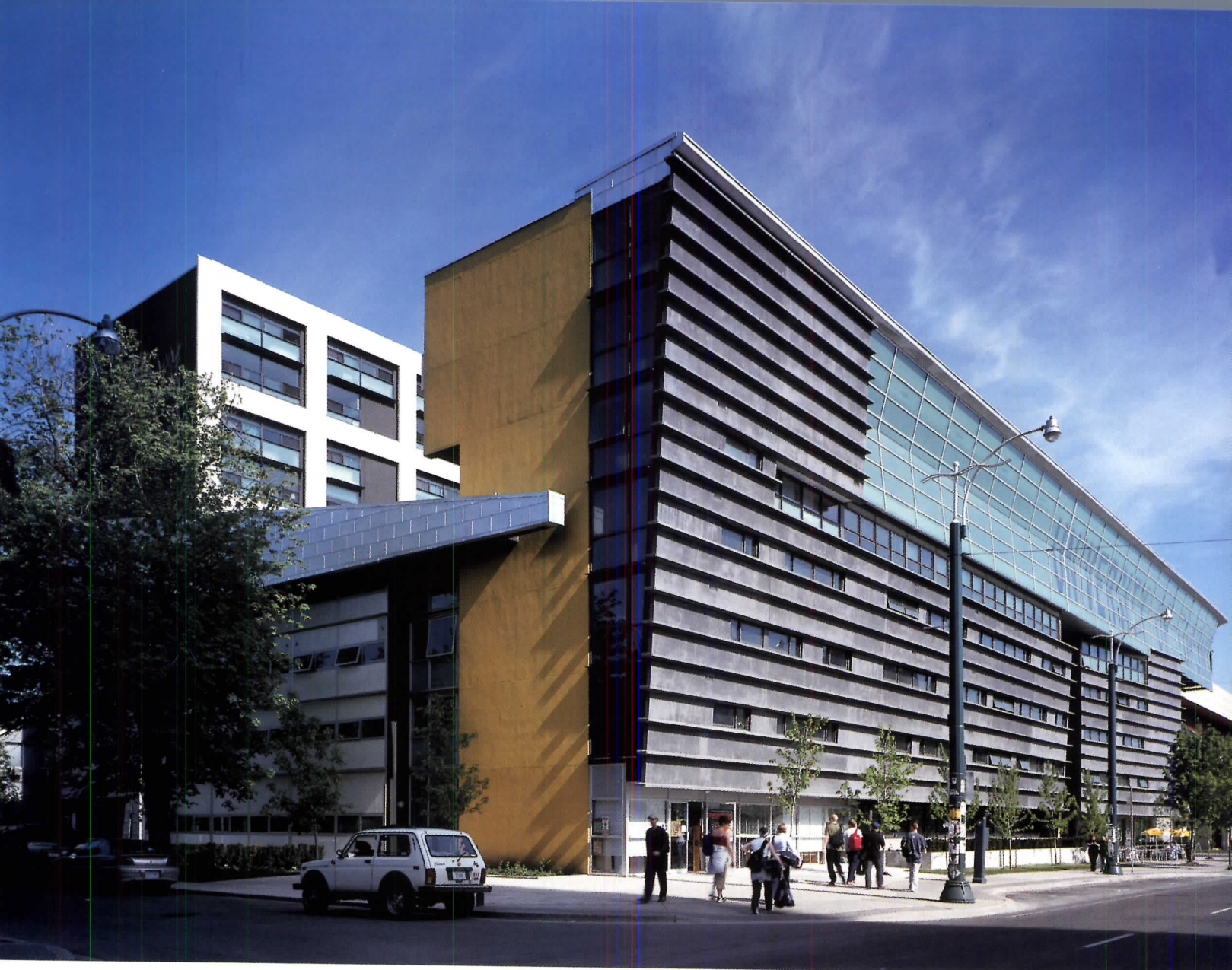
The materials and treatment of each facade vary: On the low-scale, north end (above), a mustard-tinted stucco coats the concrete shear wall, and aluminum shingles cover an abstract gable element. The ribbed concrete planks of the west facade are integrally painted a gray-brown.
