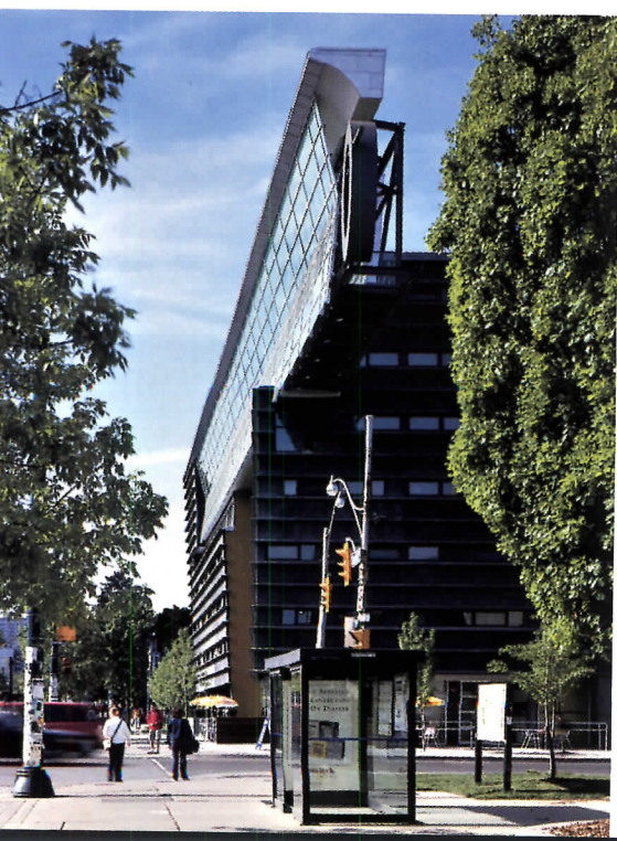
The materials and treatment of each facade vary: On the low-scale, north end (above), a mustard-tinted stucco coats the concrete shear wall, and aluminum shingles cover an abstract gable element. The ribbed concrete planks of the west facade are integrally painted a gray-brown.
