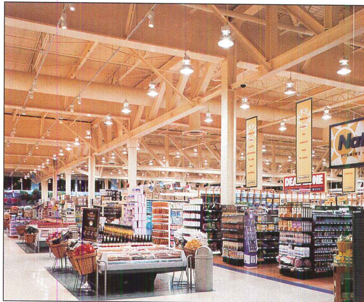
Loblaws grocery store at St. Clair and Bathurst, Toronto. ON Architect: Turner Fleisher Architects, Inc. Photo: Lenscape Inc. A/D FIREFILM® II on trusses and columns
