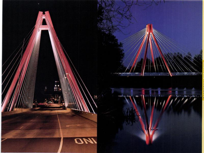
The goal of the lighting plan was to accentuate the structural design of the bridge. "Light shines up the cables in the same way as the structural load is carried," says designer Jim Baney. The superstructure is fully suspended from a single quadripod pylon by two inclined planes of 40 stays. Blue marker lights designate the juncture where each cable stay engages the bridge deck. The stays and four pylon legs are grazed from below by metal halides to emphasize their verticality.
