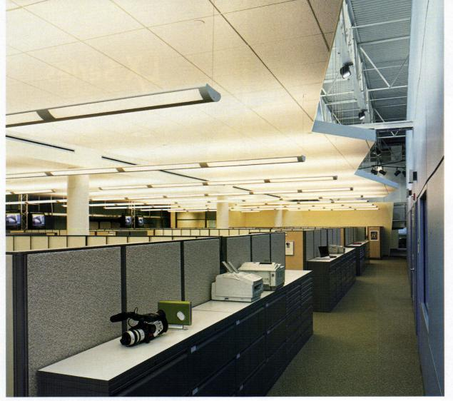
Within the second-floor office areas, runs of T8 fluorescent pendants provide both ambient and task illumination (right). Above the jagged-edged dropped ceiling, a row of metal halides washes the blue wall that encloses the broadcast television studio (right and below). Lighting works in tandem with architectural form to open the workings of the studio to the public realm.
