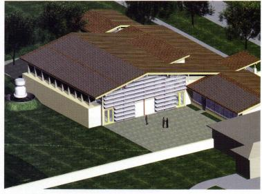
The hall roof (above) has south-facing photovoltaic panels. A chiller sits on top of a 10,000-gallon water reservoir. The interior (left) is built of recycled log columns and cedar glulam beams.
