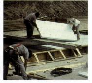
Nonconductive dowels are used to sandwich two withes of concrete and a layer of rigid insulation.
