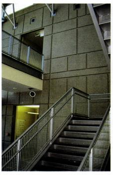
Software developer Tibco used tinted concrete and reveals in its tilt-up construction.
