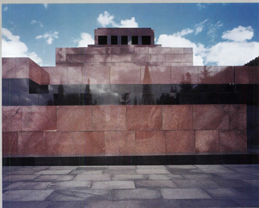
Above: The south facade of the Lenin Mausoleum by Schusev was completed in 1931. The highly polished granite facade reflects the towers of the Moscow Kremlin and the building that was until recently the Lenin Museum.
