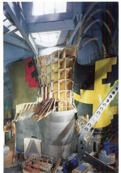
Construction of some interior elements was "paperless," with computer details going directly to fabrication.
