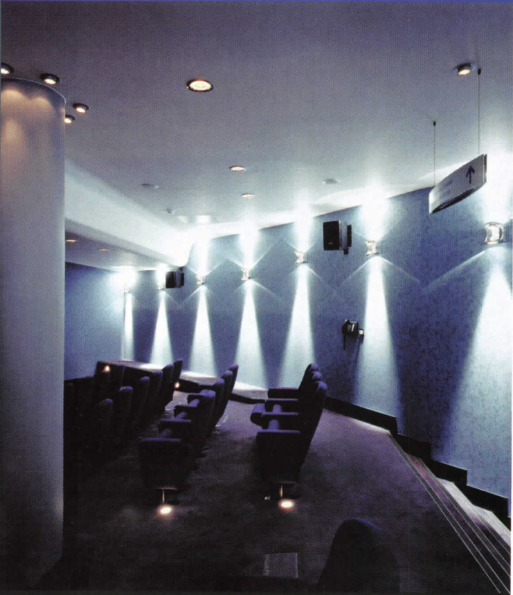
Prince. The perimeter of the auditorium (bottom right) is defined by wall sconces incorporating pairs of low-voltage QR111 lamps whose transformers have been remotely mounted. Aisles are marked by recessed uplights.
