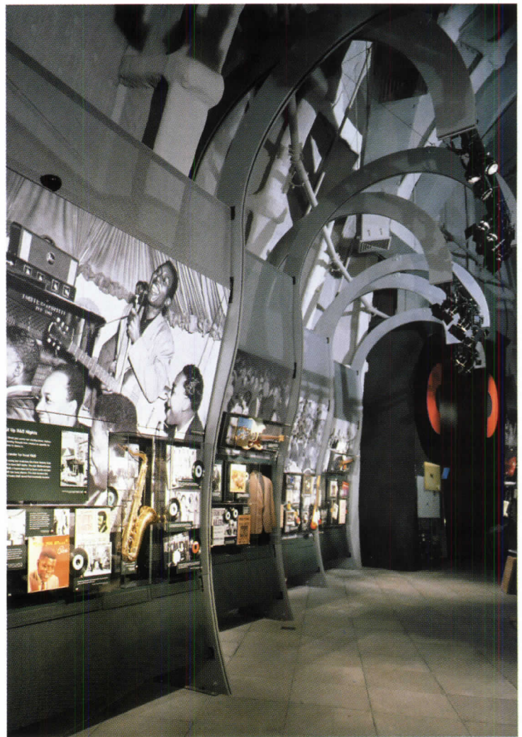
Northwest Passage, an exhibit area devoted to local music traditions, slips between the fireproofed steel ribs of Gehry's structure.
