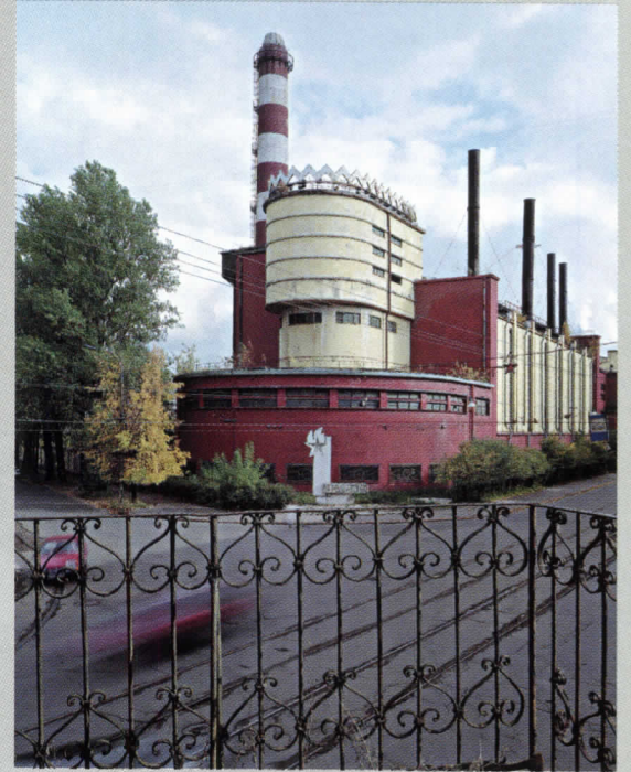
Below: Red Flag Textile Factory powerhouse by Erich Mendelsohn, St. Petersburg, 1926. The building stands in a quiet part of the city and has an almost maritime quality. The large chimney is not shown in the original model of the project.
