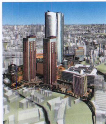
Roppongi Hills development (above) includes a 54-story curvilinear tower by KPF and Fumihiko Maki's TV Asahi Broadcasting Center (top).
