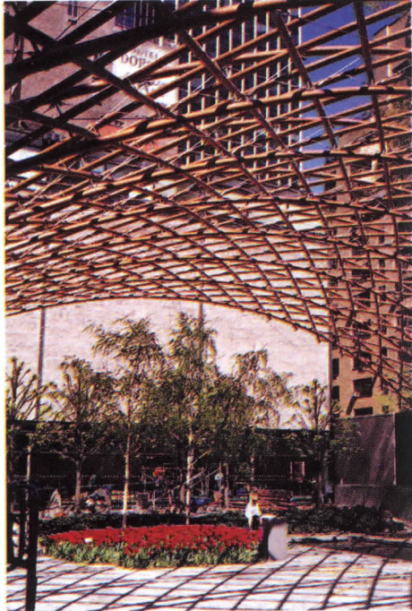
Architect Shigeru Ban's lattice arch creates dappled light in the MoMA sculpture garden.
