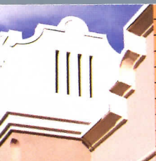
Custom coping with factory-fabricated scalloped corners in designer Kynar 500®/Hylar 5000® color.
