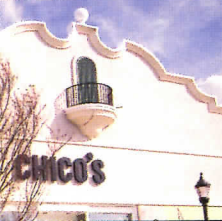
Roof-edge treatment featuring arches and inverted arches combined with serpentine, parabolic and compound curves.
