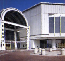
"Bullnose" profile coping rollformed to a 24" radius in .125 aluminum.
