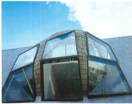
Top of the bulge: a clerestory (detail right) admits more natural light onto the rippling walls of the interior.
