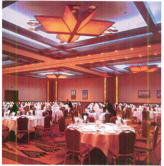
A ceiling mural is washed by uplight from 50W, 3,000K compact fluorescents mounted in side troughs (opposite). A valance
