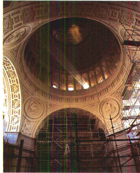
The San Francisco City Hall's dome, with scaffolding during renovation.
