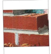
are inexpensive and easily installed in weep holes to insure masonry cavity walls breath, drain and dry quickly. Made from 100% recycled polyester with a 90% open mess in 2.5" x 4" x.5, they are available in white, tan, almond, gray, and brown. Weep Vents add to the beauty of the wall by duplicating the texture and color of mortar, thus eliminating open holes and dark shadows while restricting entry to insects. Call (800) 664-6638 for more information.
