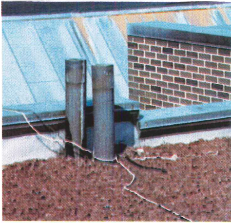
Pipe penetrations at curbs (left) are a roofer's nightmare, only made worse by the wiring. An independent roof inspector can call attention to such contrary-to-specs conditions as new roof materials stored where they can get wet (right).
