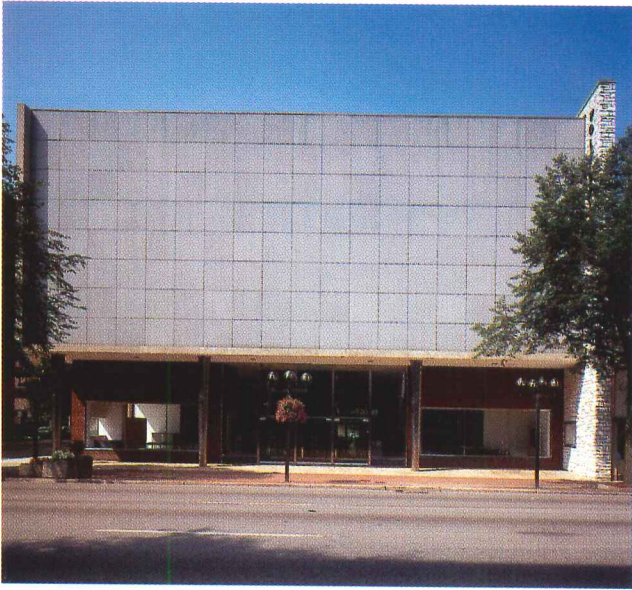
The Main Street front of the Wolf Wile store was restored (left) and a new entry for Gray was created with painted I-beams “completing” the sliced-off end of the building’s envelope (below).
