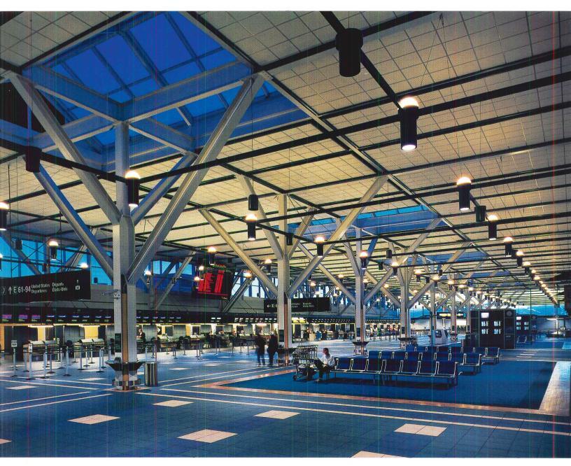
In the terminal's ticketing concourse (above), downlight cans with indirect-uplight components are suspended from steel hanger frames. In the food court (right), clusters of glass globes with compact-fluorescent lamps arch from poles reproduced from an earlier era, giving the space the feel of a seacoast village. On the skybridge, linear fluorescents hung in a chevron pattern direct passengers to customs.
