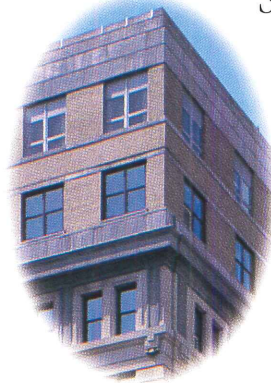
Hotel du Pont; Wilmington, DE: Clear Float Glass outboard and Energy Advantage Low-E Glass inboard; renovation project.
