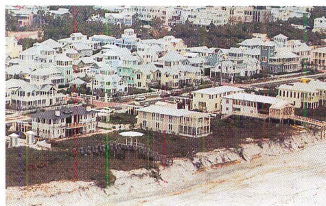
Waves up to 20-ft-high demolished ocean-front homes in Mexico Beach, Fla (top). Only a few miles away, Seaside (bottom), set behind a 100-ft-wide dune, sustained only minor wind damage.
