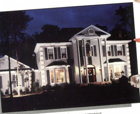
Stucco-look DUROCK exterior, residence, Mobile, AL
