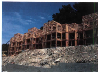
Wood-frame construction delivers cost-effectiveness in high density areas and difficult terrain.
