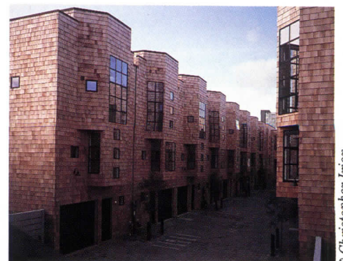
Fulton Grove’s mid-block alley was formed by joining back-to-back land parcels.
