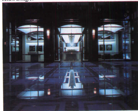
A functional indirect-lighting system in this architectural office also makes an esthetic statement. Above is the main entrance as seen from outside in the public corridor. Panels in the reception area and gallery (right), conference rooms, and partners' offices were curved as shown in the concept sketch below, but were hung flat in the design studio to reduce cost. Custom valances (fluorescent wall fixtures) designed by Allan Leibow of WGFS were introduced by the lighting designer to improve the balance of brightness in rooms such as the gallery.
