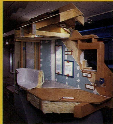
The Pacific Energy Center includes this demonstration of upgraded insulation.
