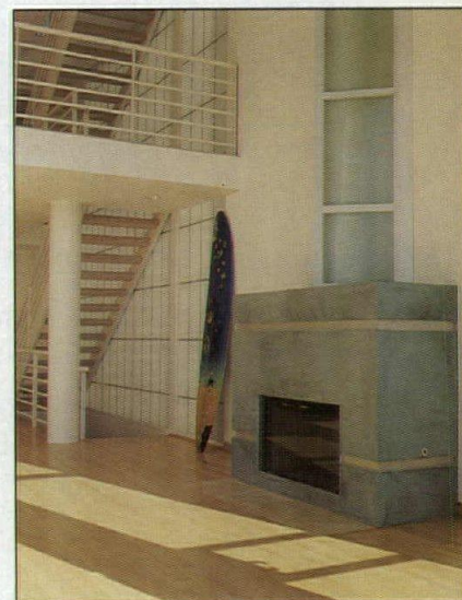
The Fry reveal pattern is continued on the interior walls and around the fireplace.
