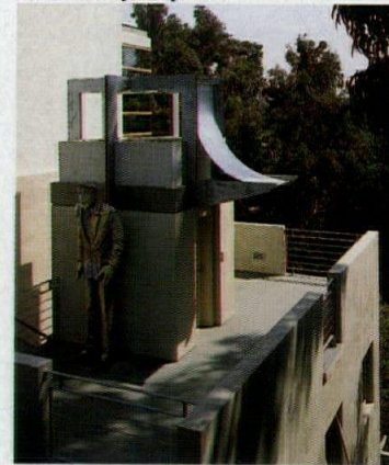
Frank Israel’s art pavilion is a box with many faces: on the street side, the poured-in-place concrete and concrete block volume presents itself with a stucco base beneath a facade of composite concrete panels framed in wood (opposite top). Trusses protruding from inside support lead scuppers. Seemingly seamless corner windows echo Rudolph Schindler. An elevator shaft repeats the composition of the main building (above). On the garden side, an arcaded walkway and balcony link the building to its site (opposite bottom).
