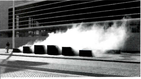
318. Fog effects. The Mee system pressurizes tap water and atomizes it into a cloud-like mist. Described as energy-efficient, installations use very little water while creating unique microclimates for zoo exhibits and botanical gardens, special fountain like landscape displays (pictured), and evaporative air conditioning that cools people in outdoor parks. Mee Industries, Inc.
