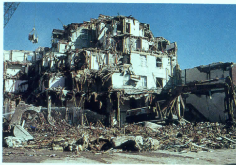
Bay Area earthquake
