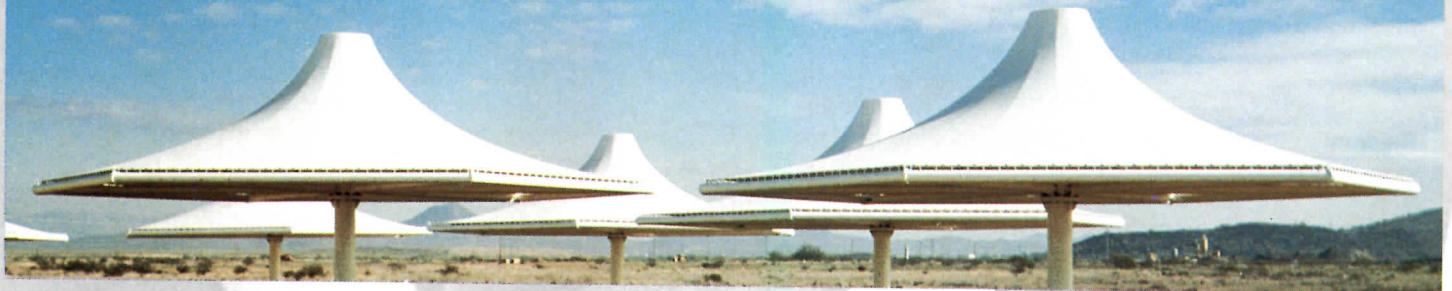
Individual Modular Shelters, Phoenix, Arizona.
