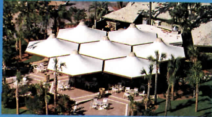
Resort dining and refreshment center, Wesley Chapel, Florida.
