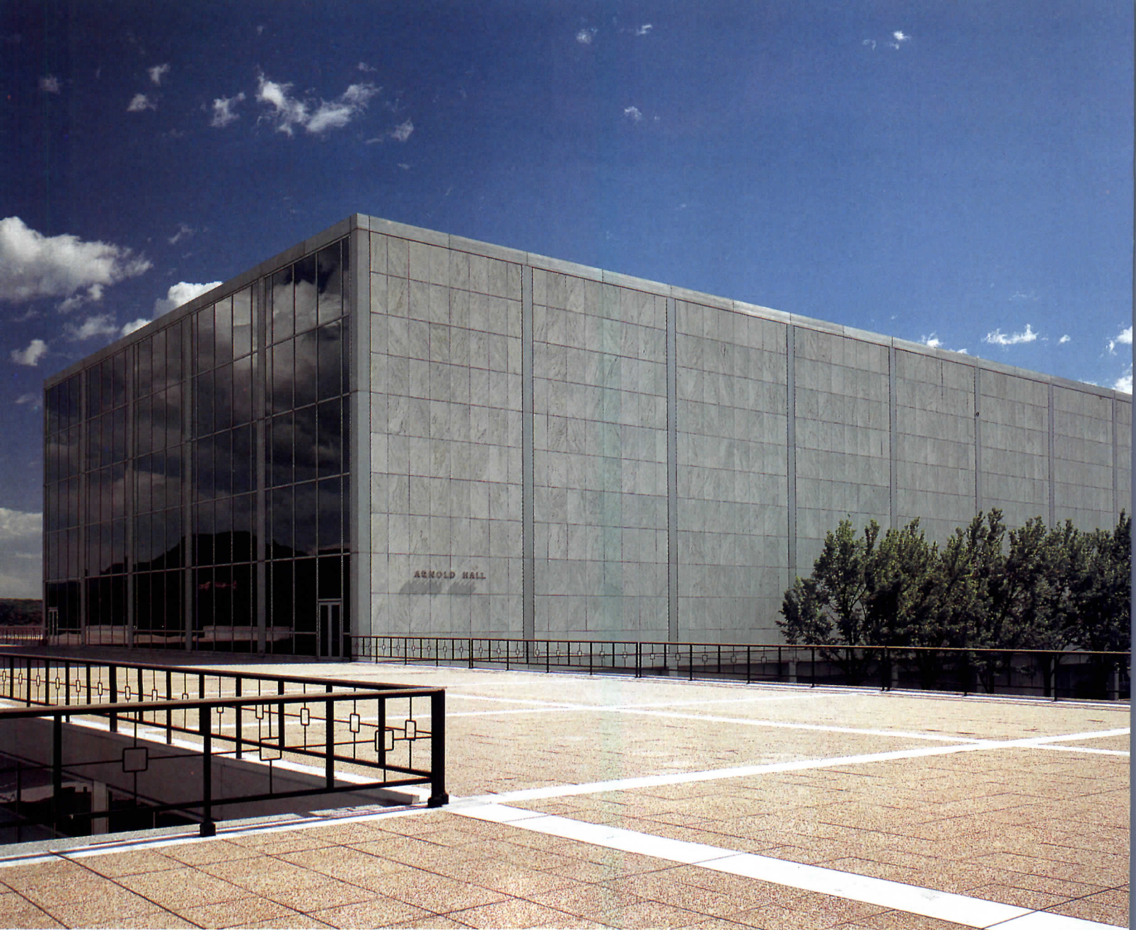
Buildings: U.S. Air Force Academy, Colorado Springs, CO / Architects: Skidmore Owings & Merrill / Marble: White Cherokee® Georgia Marble. Marble pavers also White Cherokee
