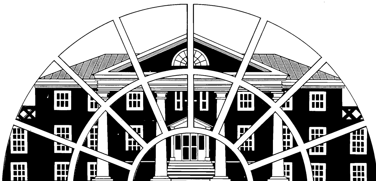
MONTPELIER, MONTPELIER STATION, VA.
