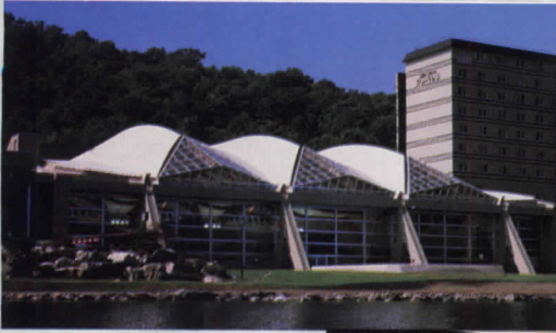
Glass gables are integrated into Sun Palace membrane roof.
