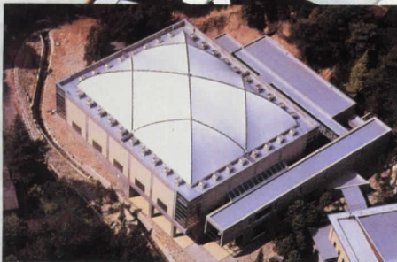
Translucent membrane roof brings daylight to college gymnasium at Hiroshima.
