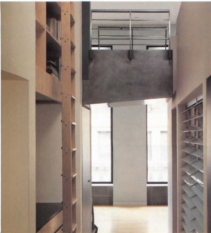
1. A cantilevered steel bridge connects master bedroom to master bathroom. 2. The staircase connecting the apartment's two levels features bowed, stainless-steel handrails that echo the curved volumes in the apartment. 3. View from the master
