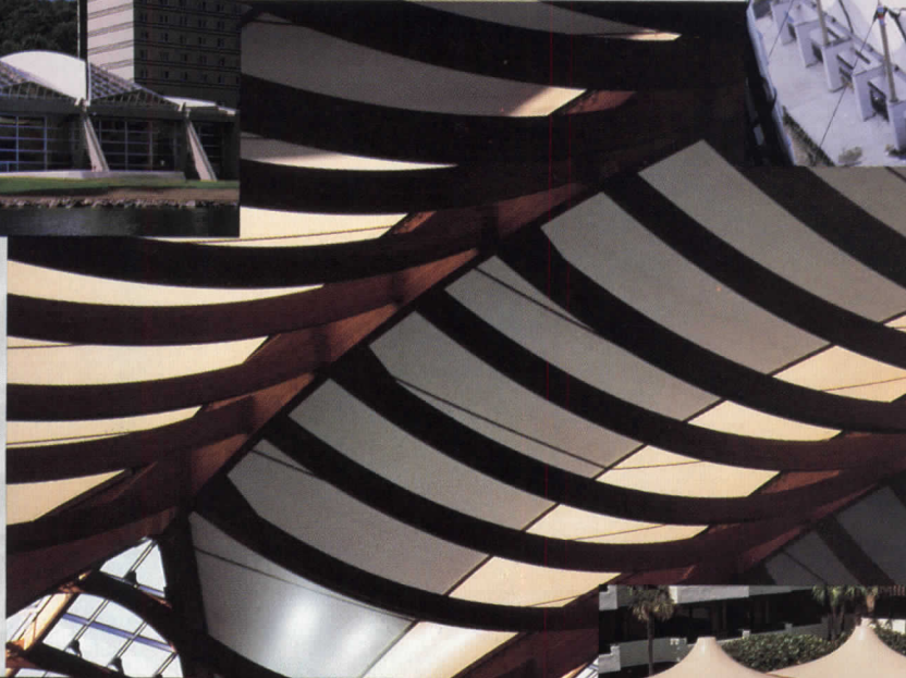
Point-hung tensioned membrane structure at Toyohashi.
