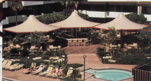
Clustered tension membrane Modular Shelters, Pompano Beach, Florida.
