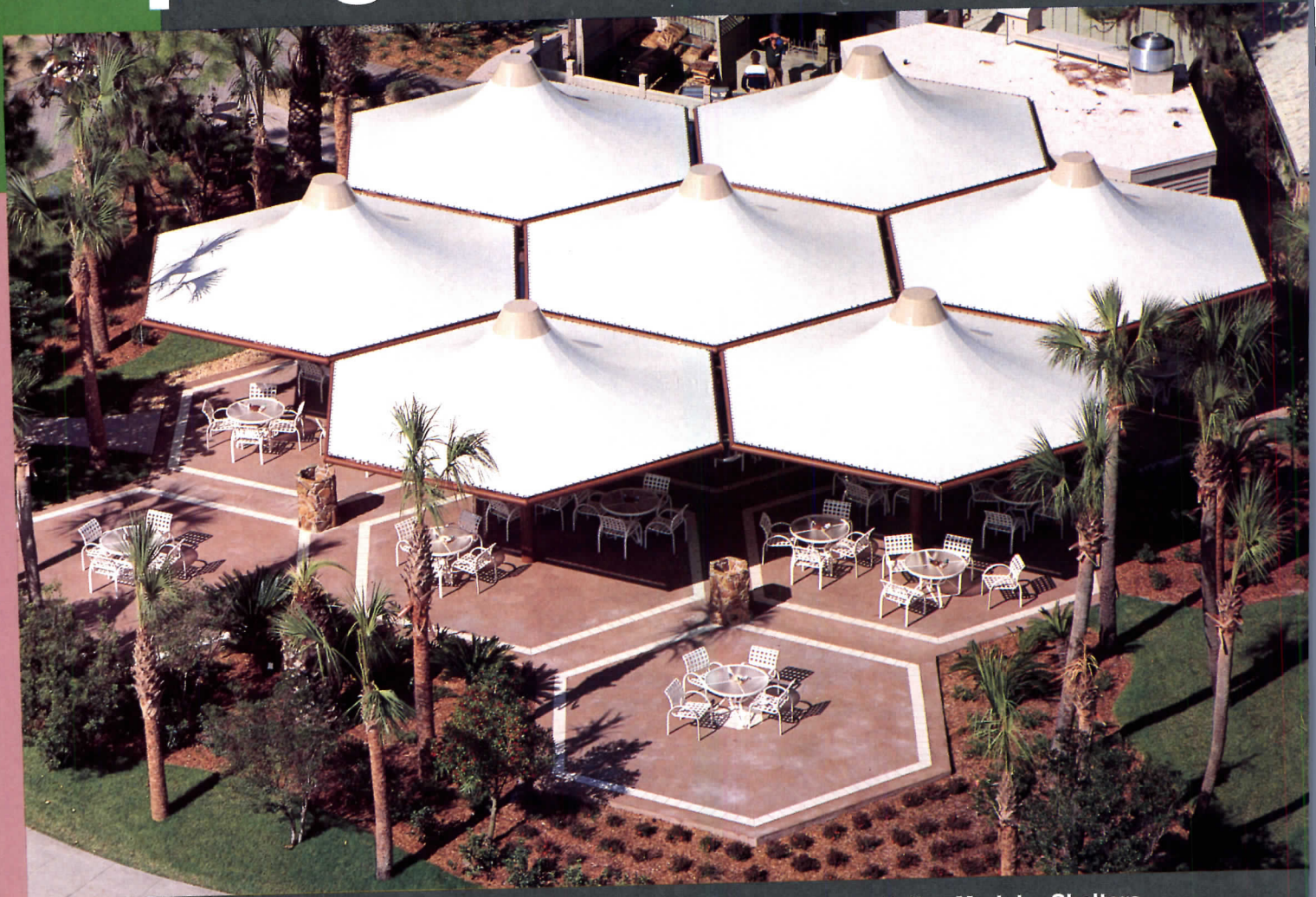
Helios Modular Shelters at Saddlebrook, Wesley Chapel, Florida U.S.A.
